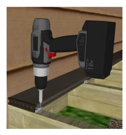
Be sure that the drill is angled approximately 90° to the solid joist when attaching the hidden clip. Be sure the clip is pushed snug to the deck board, then fasten to the joist.
