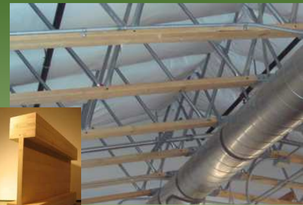
Cold formed steel & pin webs
